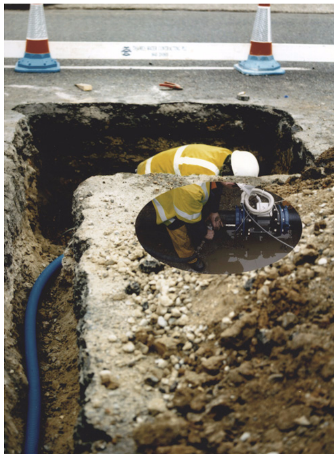
Underground Installation of MagMaster
