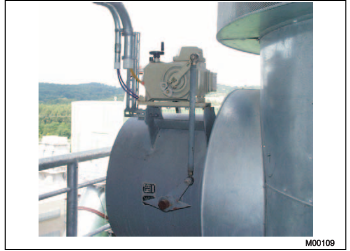
Fig. 38: Milling air control; rotary actuator RHD250 (rated torque 250 NM)
