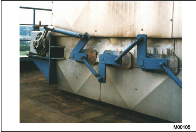
Fig. 34: Controlling exhaust gas using a rotary actuator on a multi-leaf valve
