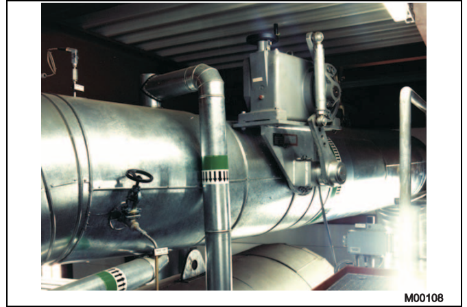
Fig. 37: Rotary actuator (air control)
