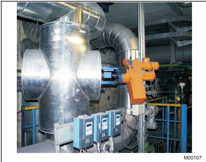
Fig. 36: Horizontally installed linear actuator (air control)
