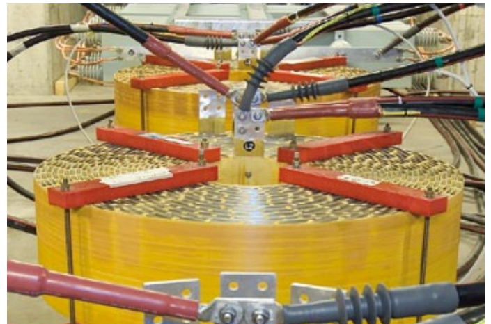
View of the test filter installation
