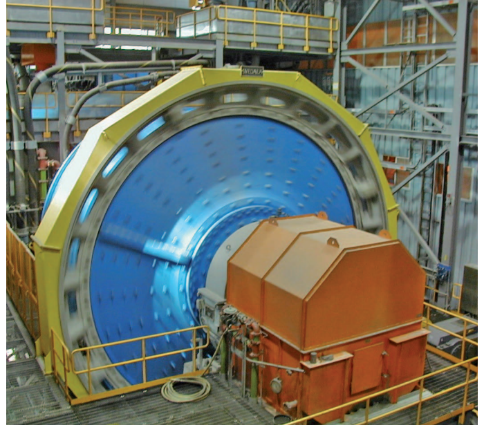
View of the SAG mill (3,360 kW) at Agnico-Eagle's LaRonde mine.
