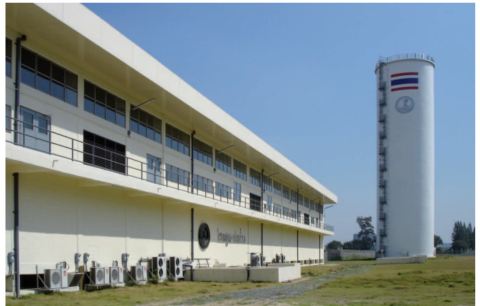
MWA's Bangkhen water transmission plant and water tower
