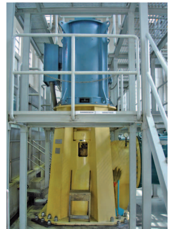
Raw water intake canal and vertical motor and pump at MWA's Mahasawat plant
