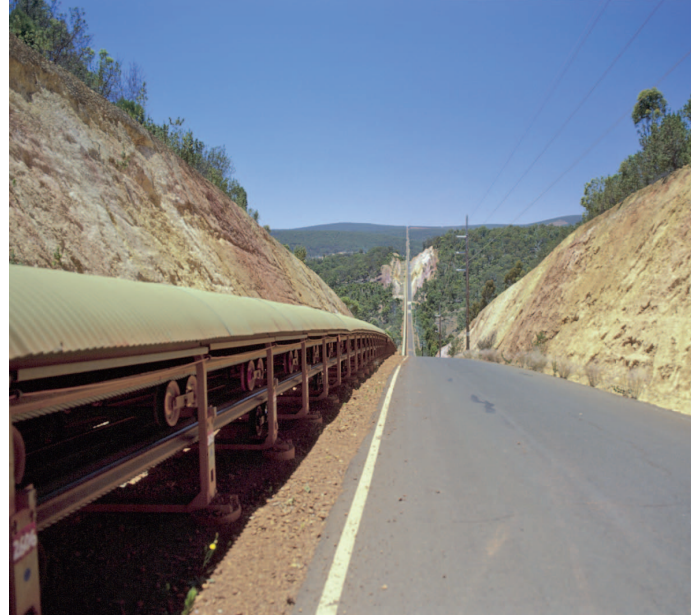
View looking along a section of the 51 km long conveyor belt.
