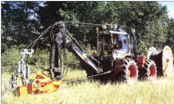
Fig. 5 shows Cable installation
