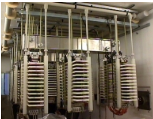
Fig. 4: Converter valve assembly.
