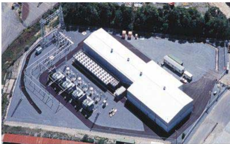
Figure 3. Cross Sound Cable, Shoreham converter station, 330 MW, aerial view. Building dimensions are 80 x 25 x 11 m (L x W x H).
