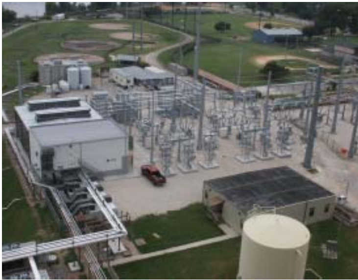
Figure 8. VSC based Statcom in Austin City Center.
