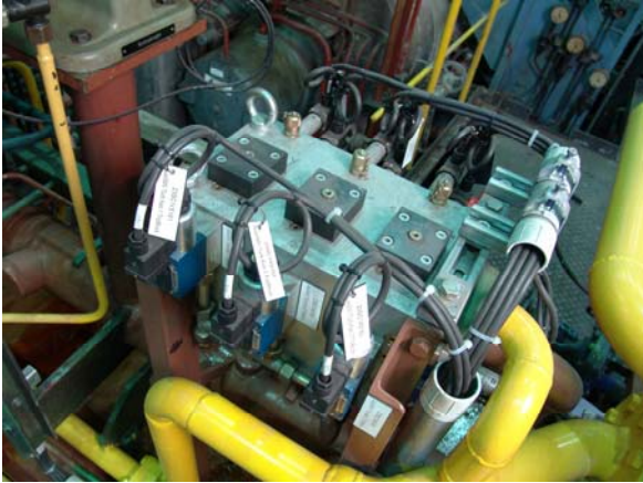
SIL3-certified 2-out-of-3 trip unit
