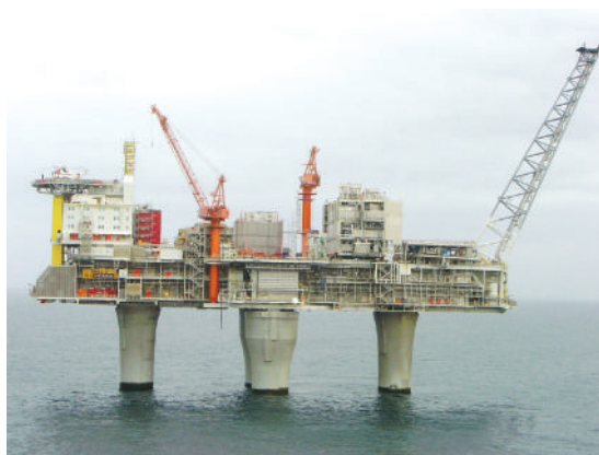
Troll platform (the HVDC Light module is seen in the middle)
