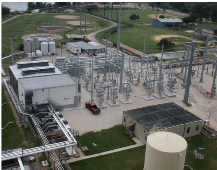
Figure 9. VSC based Statcom in Austin City Center.
