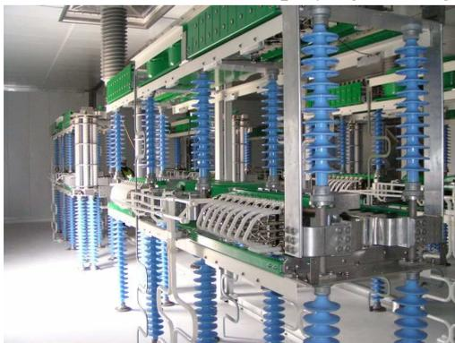
Picture 1 Inside a valve enclosure
