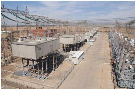
Picture 3 The Apollo station with new outdoor thyristor valves
