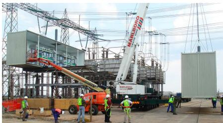
Picture 2 Installation of bridge 3 while bridge 5 and 7 is in operation
