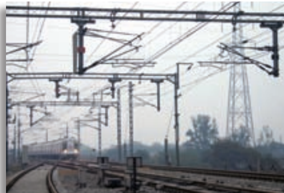
25kV AC Flexible Over Head Electrification
