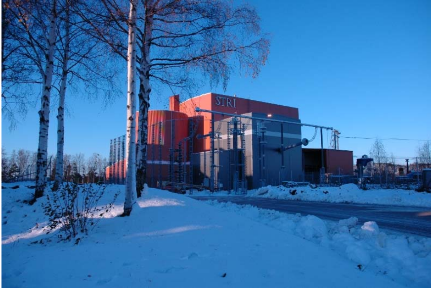
Fig. 2. 800 kV UHVDC long term test circuit installation at STRI, Sweden.
