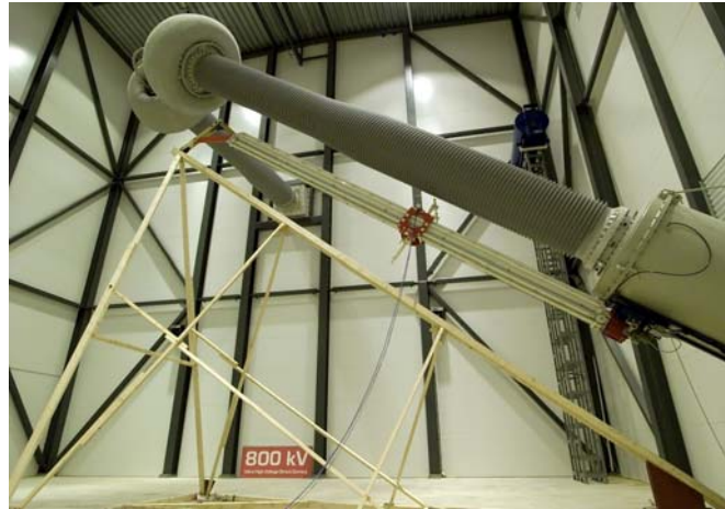
Fig. 10. Measurement of 2-dimensional DC electric field along transformer the bushing, during the long duration test. The wooden structure is used to put the robot in parallel with the bushing. The position of the probe is indicated by the red circle and it is remotely moved along the bushing..
