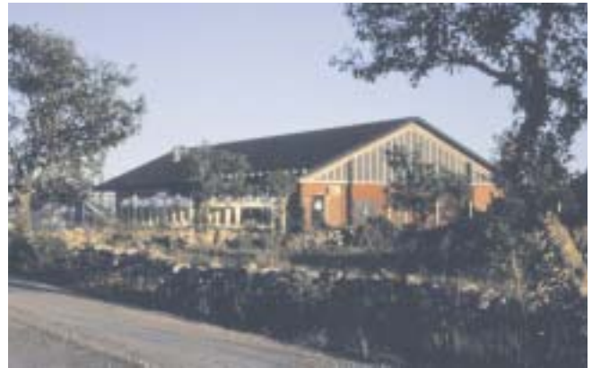
Gotland HVDC Light® converter station, Sweden
