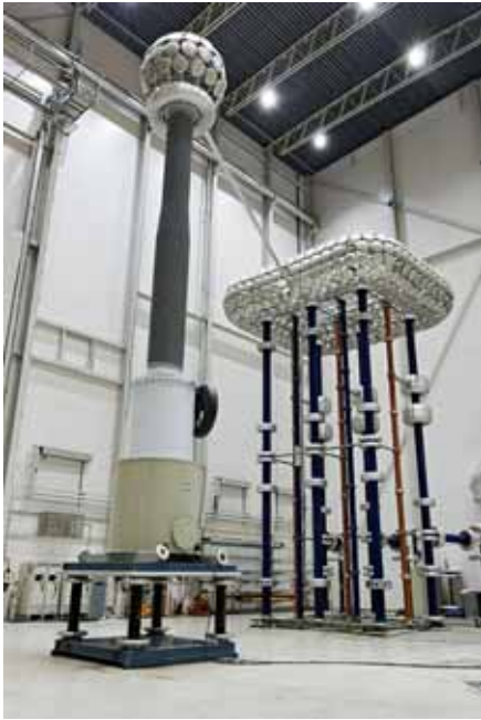
Transformer bushing testing
