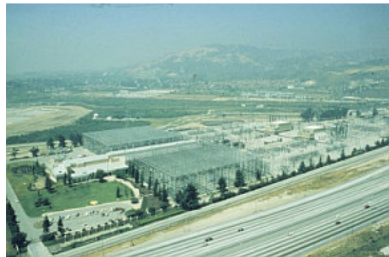
The Sylmar station in Los Angeles
