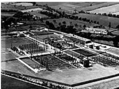
The English Channel HVDC transmission 1961. Echinghen station, France.
