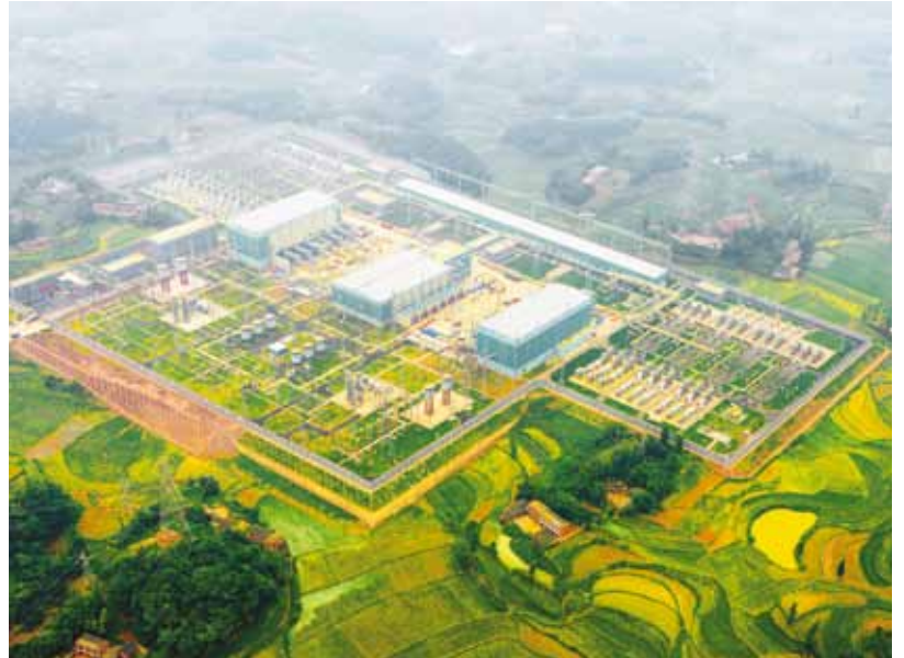
The sending HVDC station at Fulong, in south-central China
