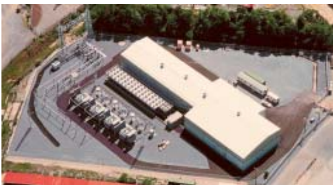
Figure 9. HVDC Light® station at New Haven
