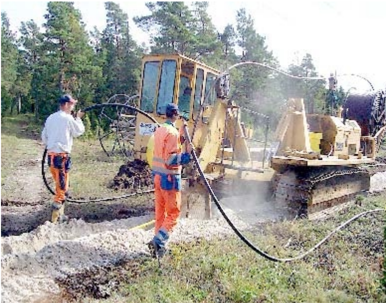
Fig. 5 shows low cost installation with plowing
