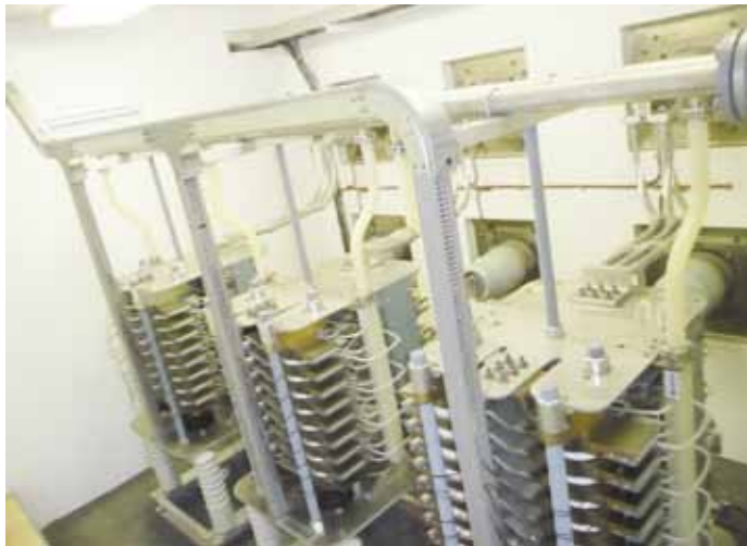
Fig. 3: Thyristor valve.
