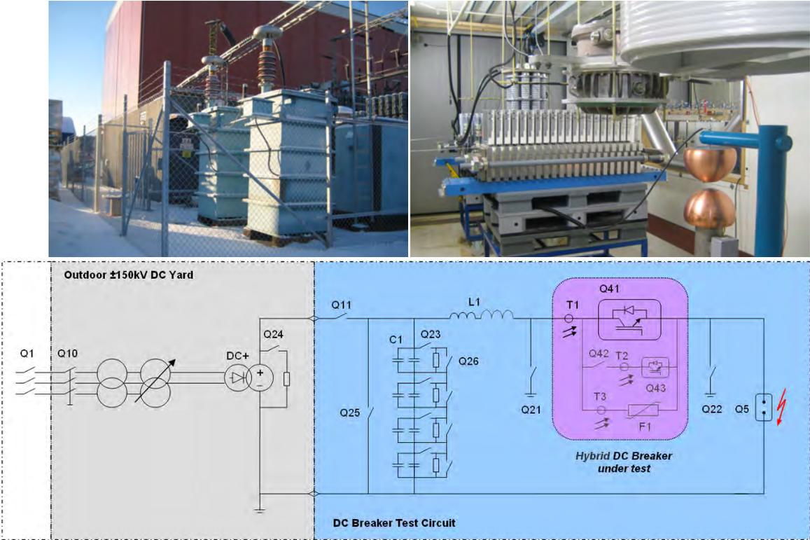
Figure 7: Containerized DC Breaker Test Circuit at ABB Ludvika, Sweden
