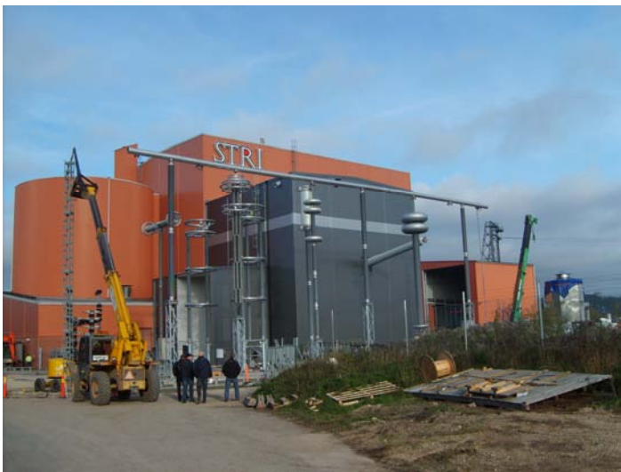
Figure 12: Test circuit during installation
