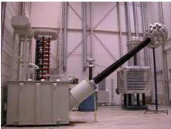
Fig 3. transformer prototype in the test laboratory
