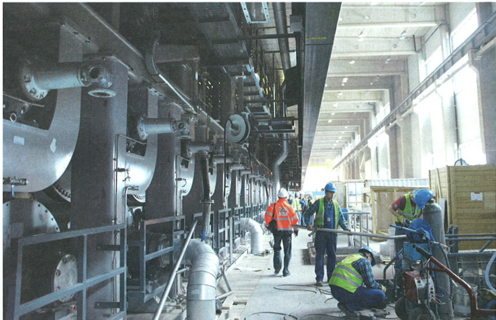
The drying section of the paper machine
