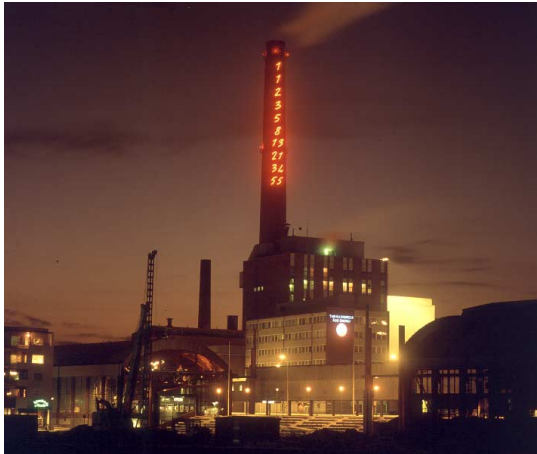
Figure 5. Turku Energia delivers electricity and heat.
