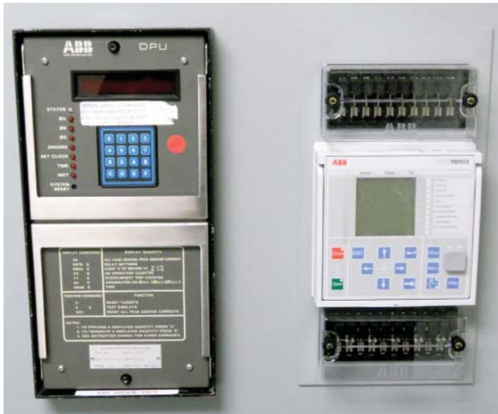
Retrofit assembly fits into the existing cut out with adapter plate.
