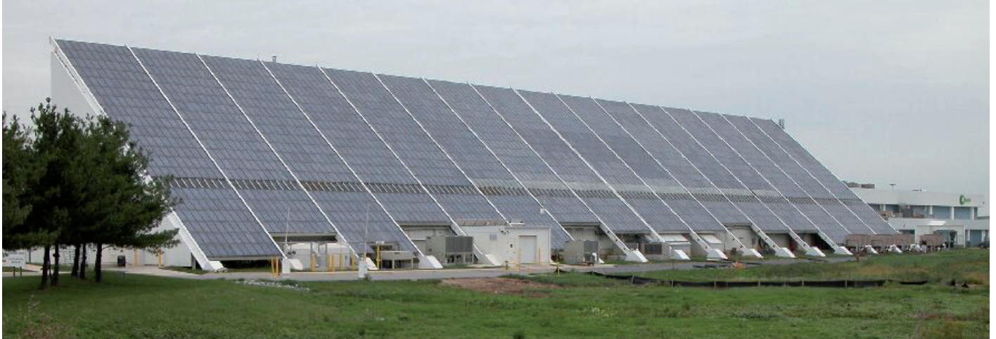
The company advertises its products on the roof on its Maryland facility
