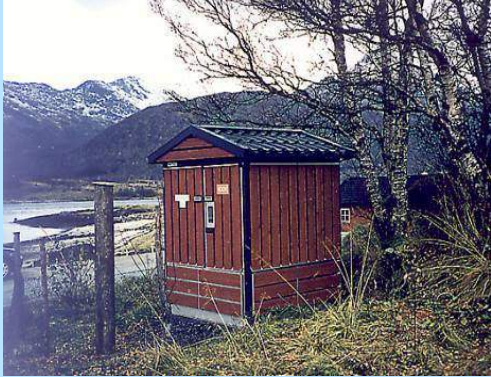
Compact secondary substation
