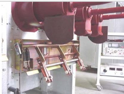
Esw in open position
