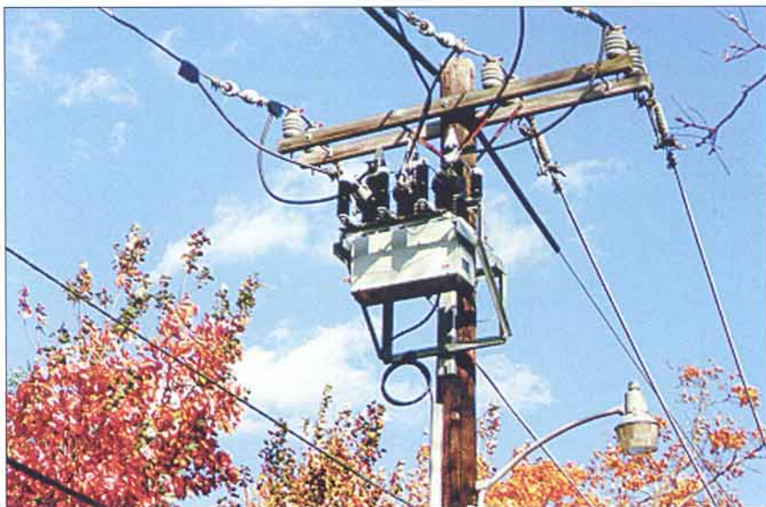
The 15 kV VR3S poletop recloser is an example of a new generation of automation-ready devices
