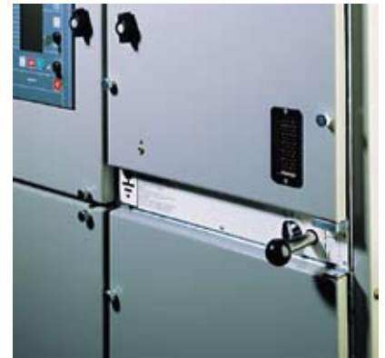
Contactor truck drive mechanism.
