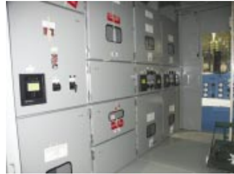
Outdoor, single row walk-in enclosure. Front aisle provides space for convenient operation and inspection protected from weather. Shipping section includes assembled aisle, minimizing field installation work.
