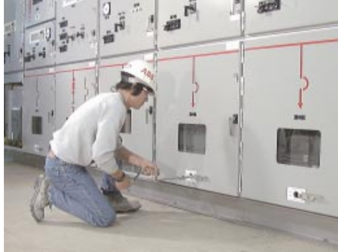
Operators are protected by the closed door racking system.
