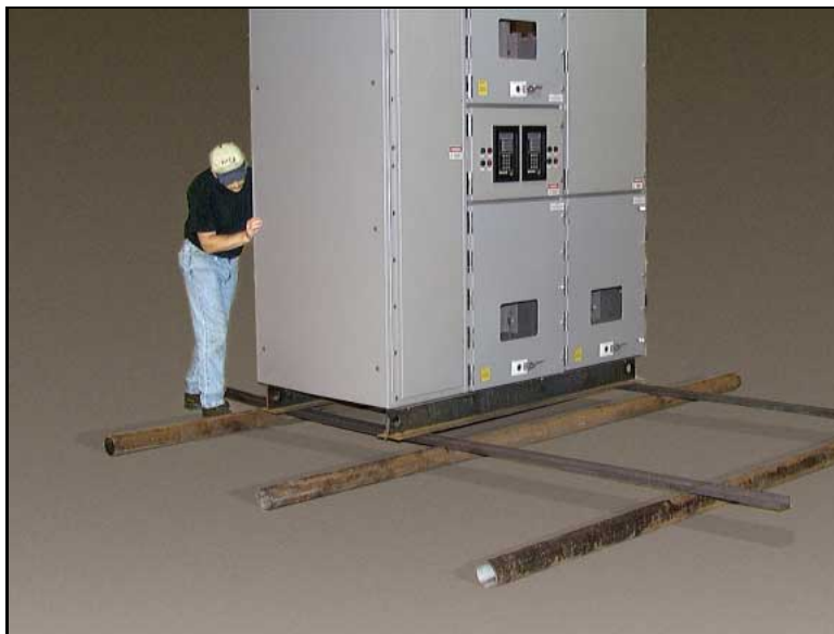
Figure 7. Carefully push the unit onto a third roller.
