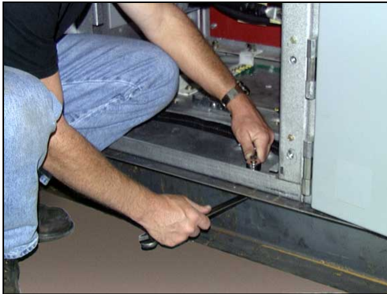
Figure 9. Unbolting the shipping base.
