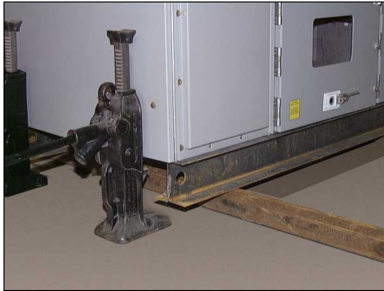
Figure 4. Insert rollers under shipping base.
