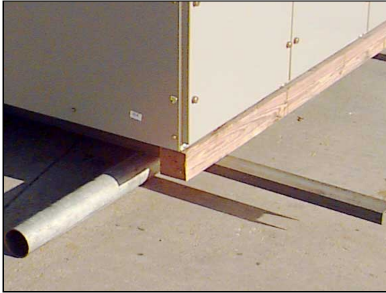
Figure 6. Position rails on rollers as shown for lateral moving.
