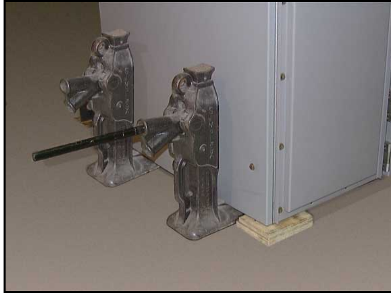
Figure 10. Remove jacks after lowering unit onto pieces of wood.
