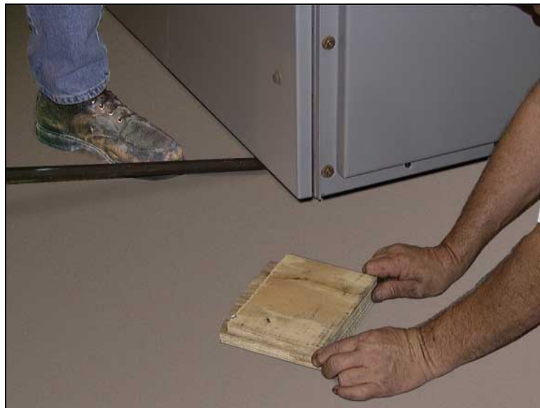
Figure 11. Use a pry-bar to remove the pieces of wood.
