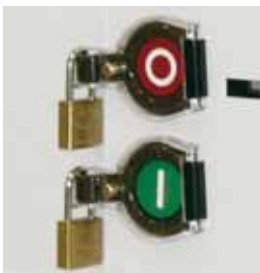
Opening and closing pushbutton locks.
