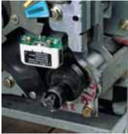
Spring charging geared motor.
