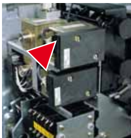
Undervoltage release.
