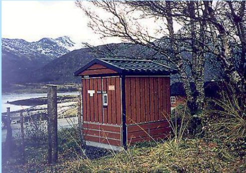
Compact secondary substation
