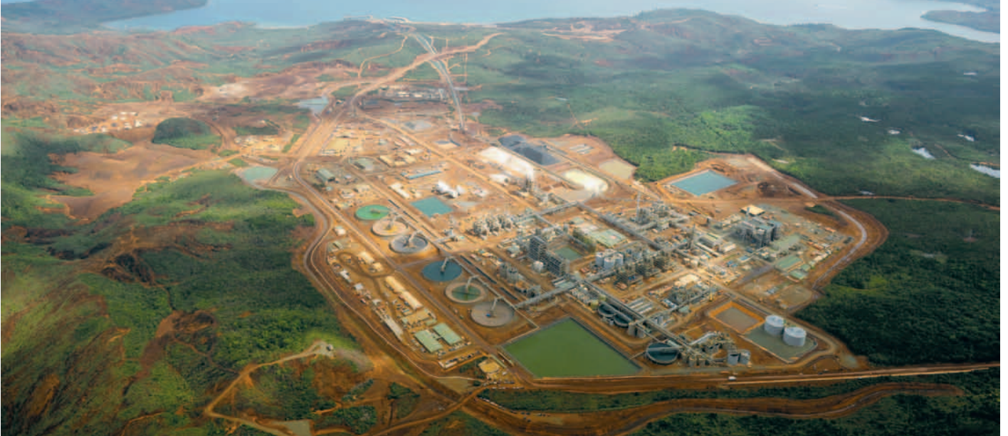
Vale Inco's New Caledonia nickel and cobalt plant
