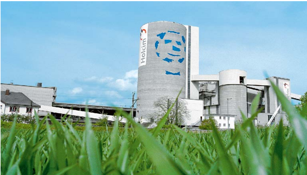
Figure 1: Holcim Untersiggenthal Plant, Switzerland, where ABB has delivered electrification, drives and optimization equipment
