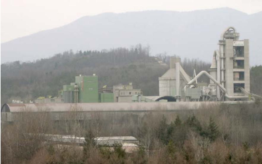
Figure4: Holcim Ternate Plant, Italy, where clinker production was increased by as much as 8% and frelime standard deviation reduced by 25% by the use of Expert Optimizer.
