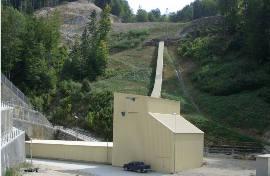
Figure 10. Downhill section, Vigier Cement Plant, Switzerland, equipped with ABB AFE technology, regenerating annually 800 000 kWh back to the grid
