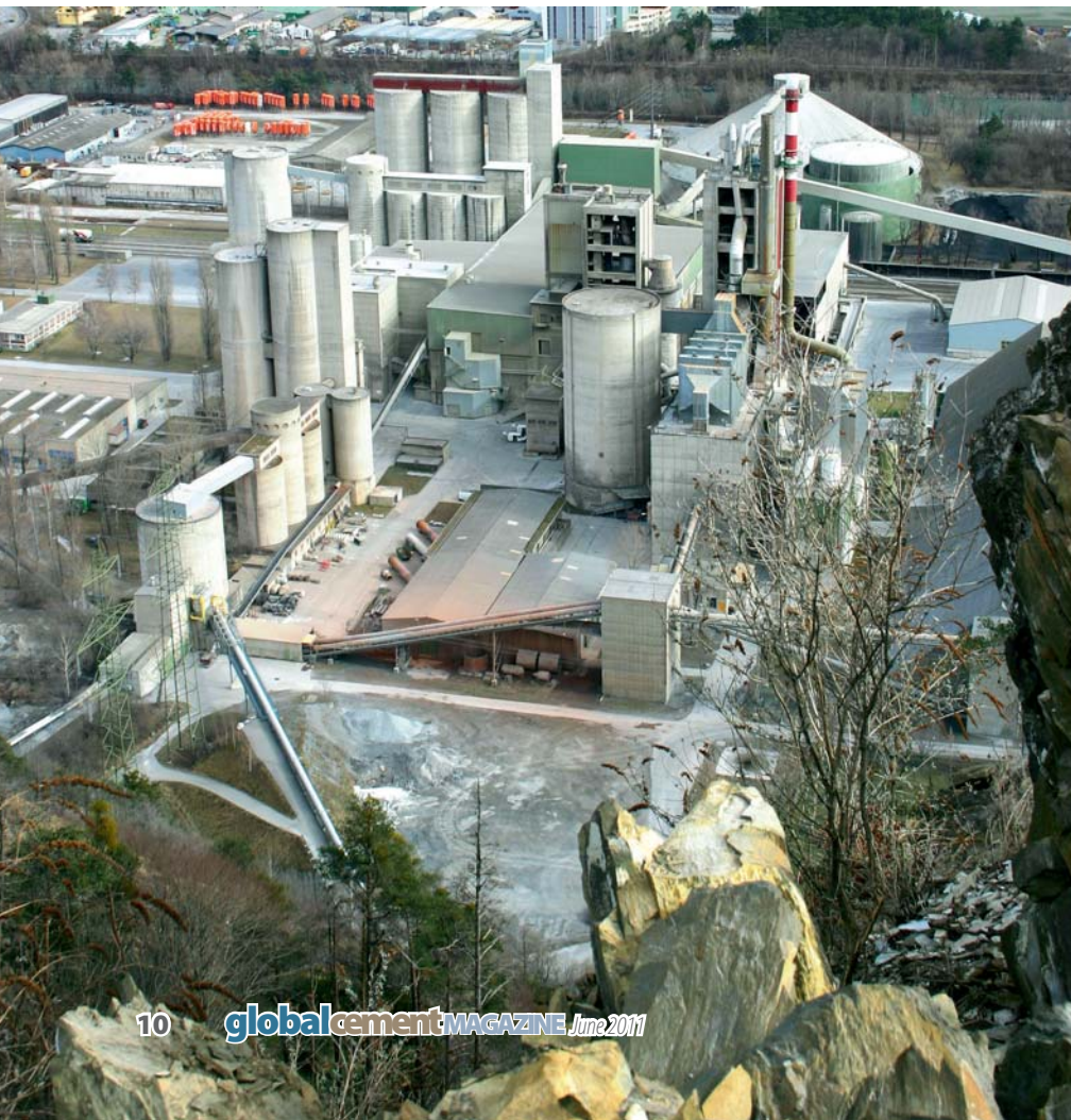
Below - Figure 2: The cement plant at Untervaz, Switzerland.
