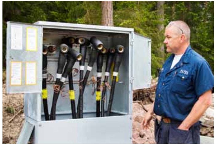
Eitel Networks like the margin of safety provided by the cable cabinets and cable connectors being touch-proof.
