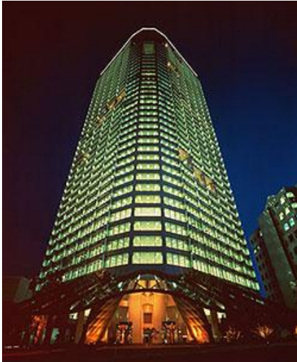
Fig. 22: Building where Power Quality problems used to lead to regular elevator breakdowns
