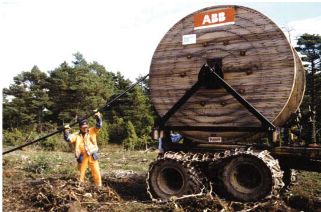
HVDC Light cables are manufactured at Karlskrona. They are then transported on drums to the location where they are to be buried in the ground. The picture above shows the first HVDC Light cable, which was installed on Gotland as early as 1999.
