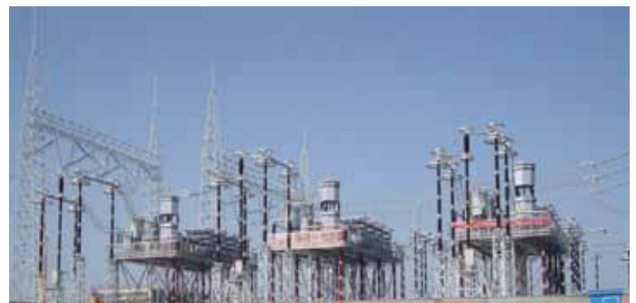
Figure 4 Series compensation for 1100 kV in China
