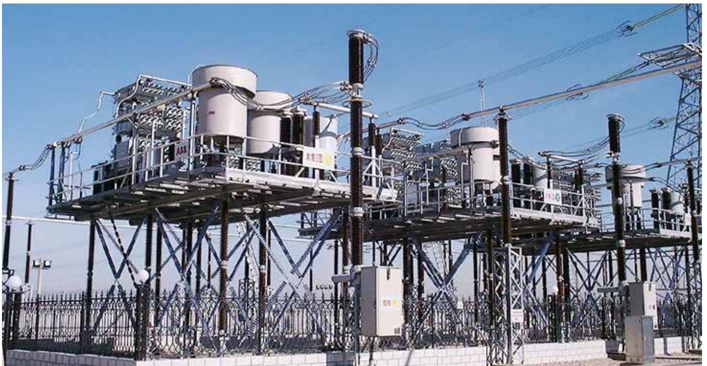
Figure 6 ABB FACTS Series compensation at Dafang, China.
