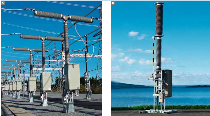
4 Disconnecting circuit breakers with two a and one b breaking chamber
