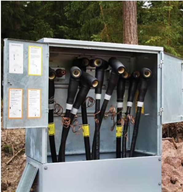
Kabeldon cable cabinet for 36 kV.
