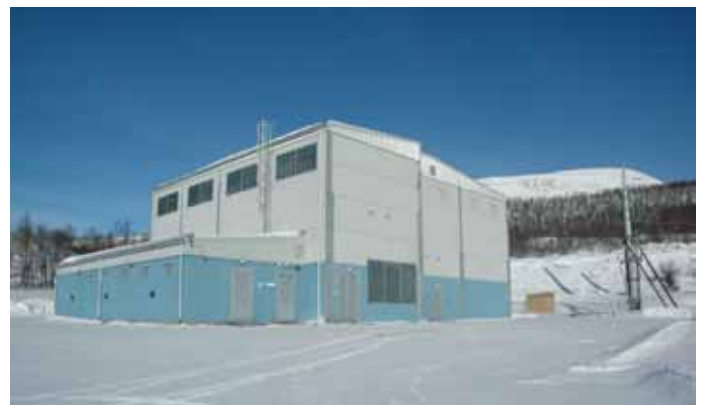
Figure 8. Example of 145 kV indoor substation with DCBs.
