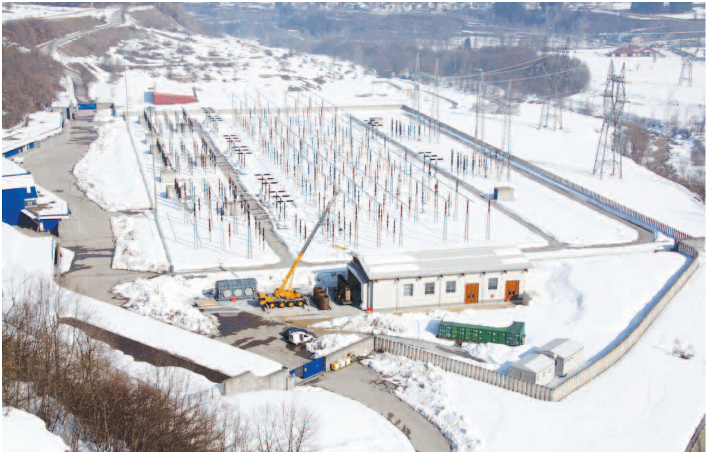
Transformer repair at the Entraque Hydro Power Plant in Italy
