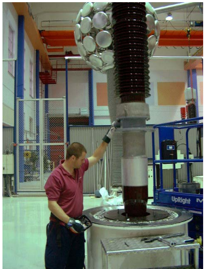
Routine testing of a 420 kV bushing type GOE(2).
