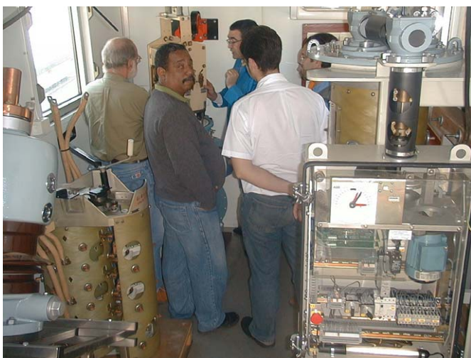
Demonstration in the container.
